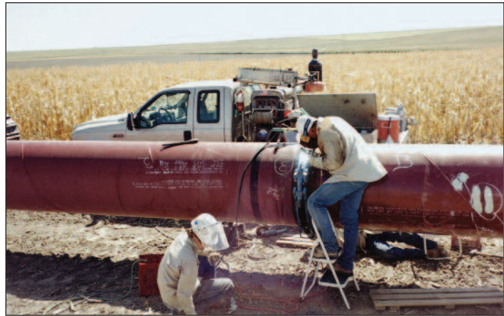
Cross-country pipe welding.
